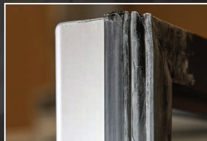
Gasket Deterioration
